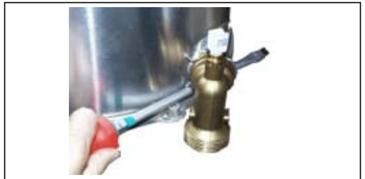
Releasing heat exchanger from the condensate pan
