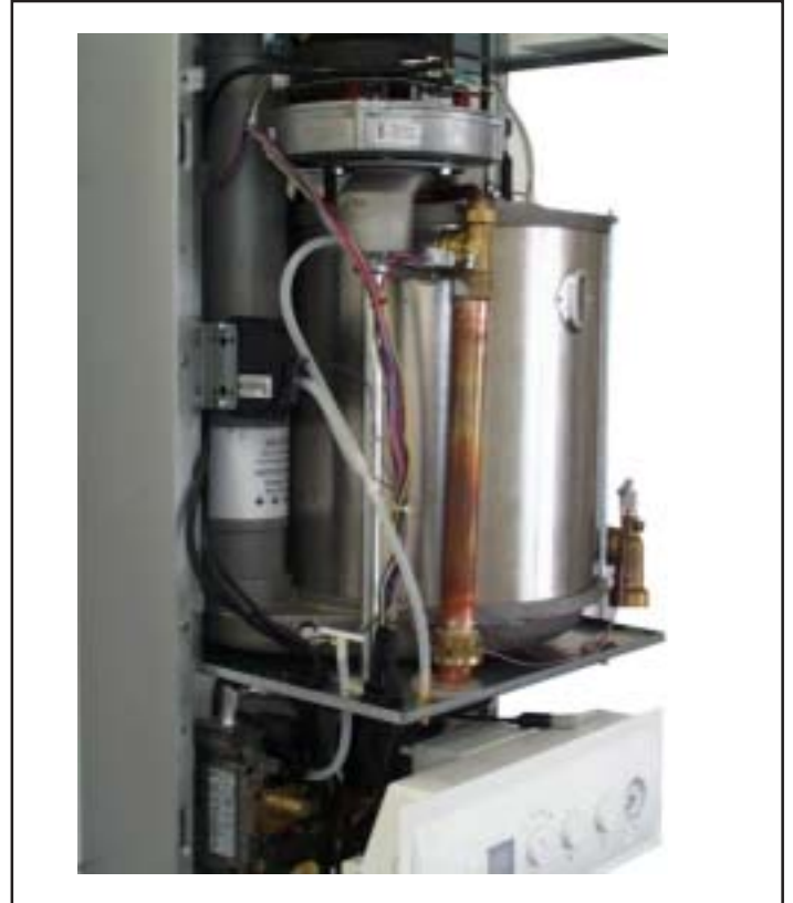
Pneumatic control cable position
