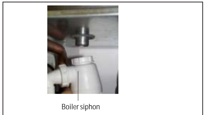
Location of boiler siphon
