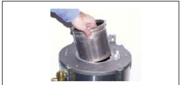
Remove the burner upwards
